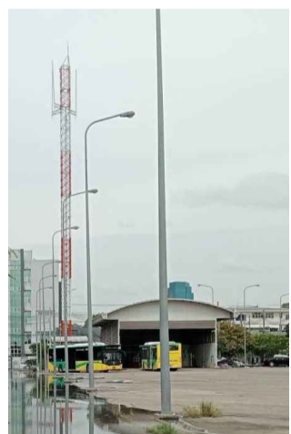
Relocate all street light poles
